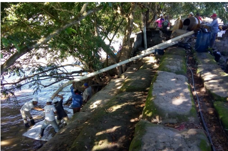
Building a flood-prevention wall in El Amparo.
